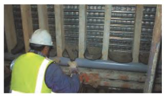
✓ If excess grout builds up on the walings and supports it is good practice to lightly brush these clean before the concrete hardens.
