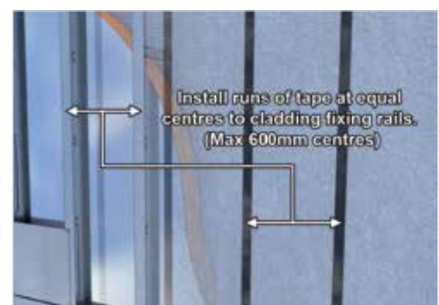
Temporary fixing
